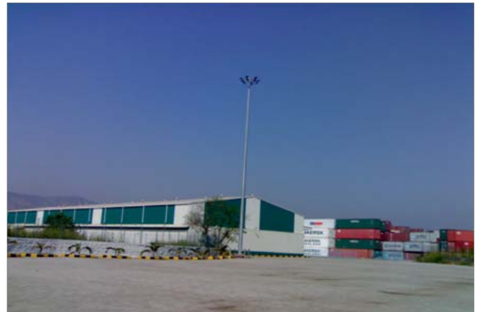
Picture2: Overview of the facility
